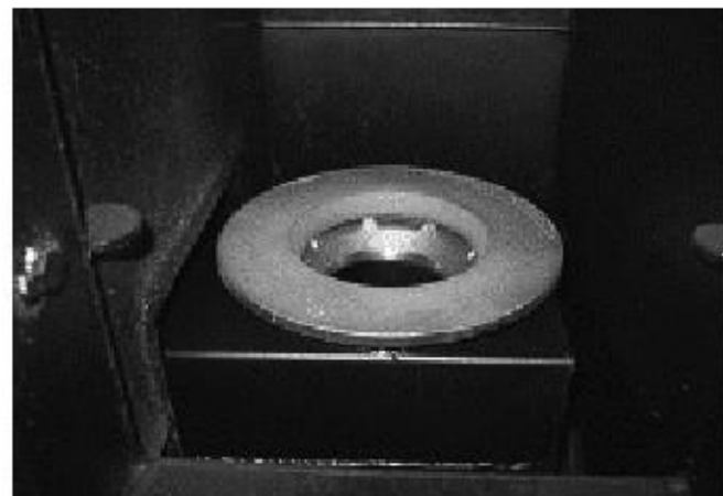
Fig. 14 Very clean combustion chamber.
