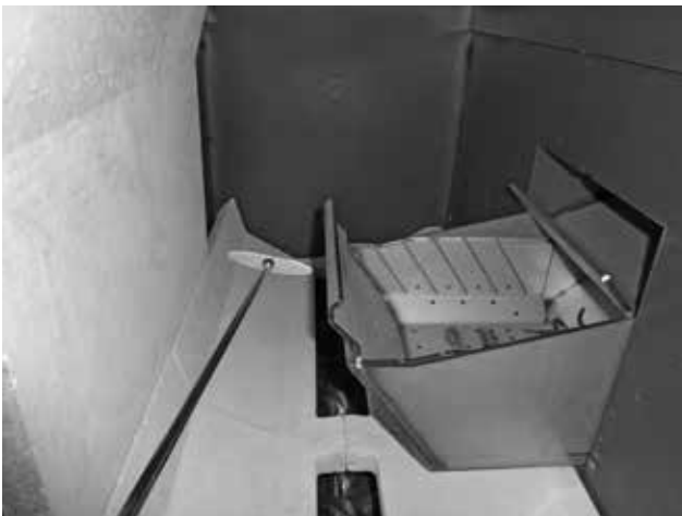
Sweeping ash into the bottom space (ash pan)
