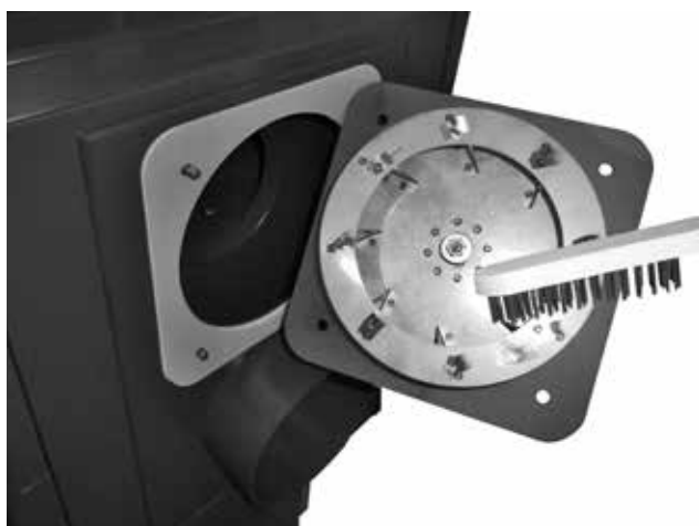
Sample cleaning of impeller on exhaust fan
