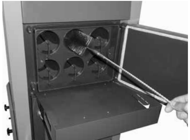
Cleaning of the tube exchanger
